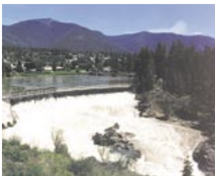
A radio receiver mounted on the Thompson Falls Dam tracks trout that are tagged with radio transmitters.
