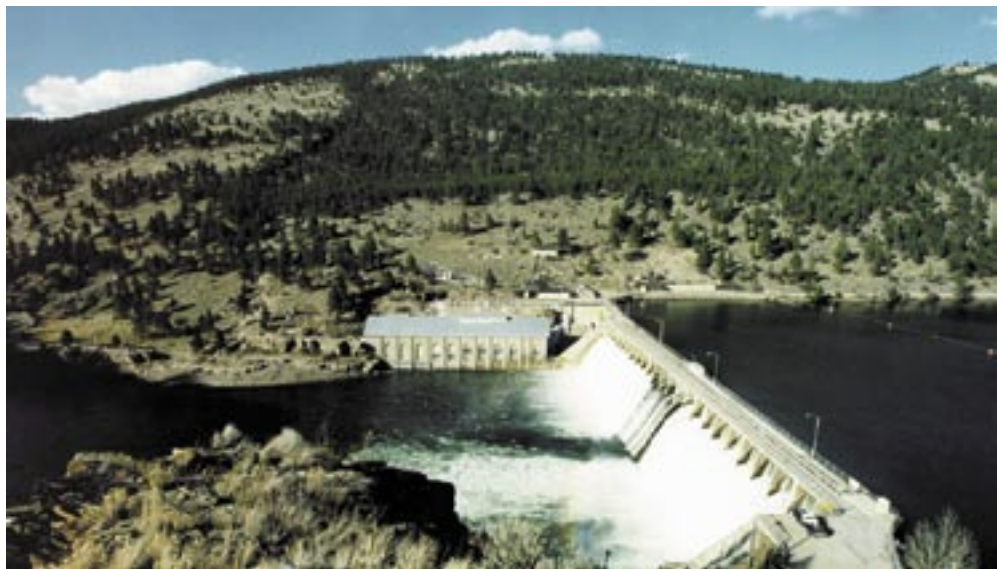
PPL's Hauser Dam, northeast of Helena, is one of seven PPL dams along the Missouri River.
