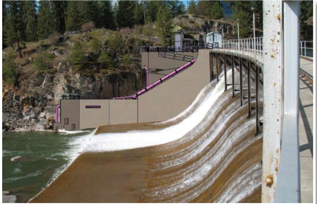
Artist's rendering of the proposed Thompson Falls fish ladder (background) in the main channel of the dam.
