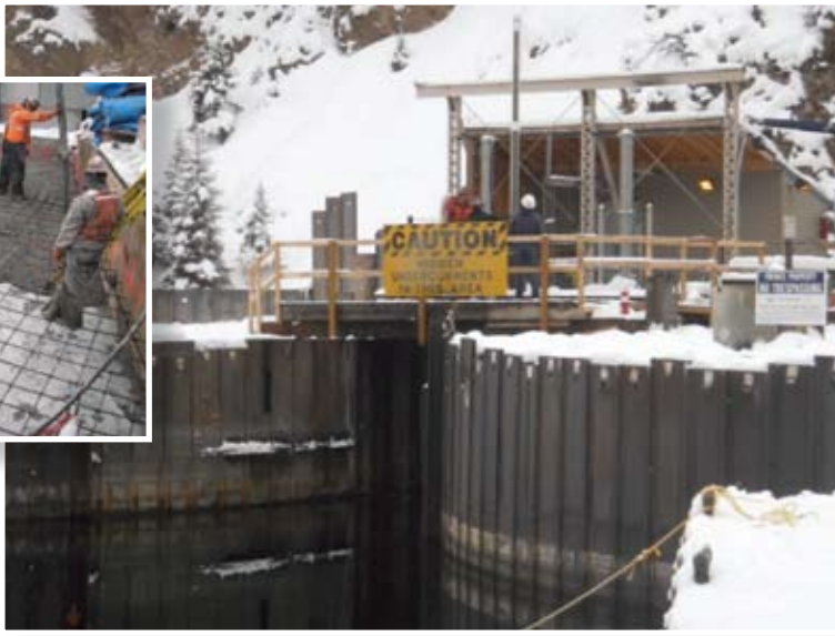
Cofferdam at Hebgen dam takes shape.
